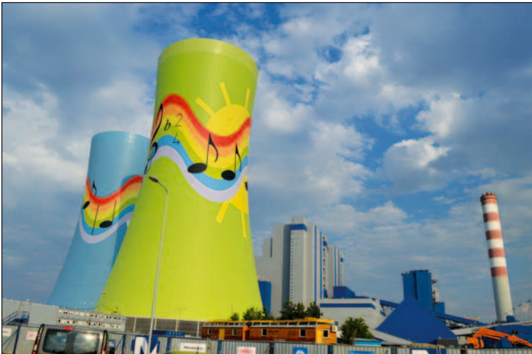
The Opole Power Station, new cooling towers, photo by Mirosław Marczyk, 2018
