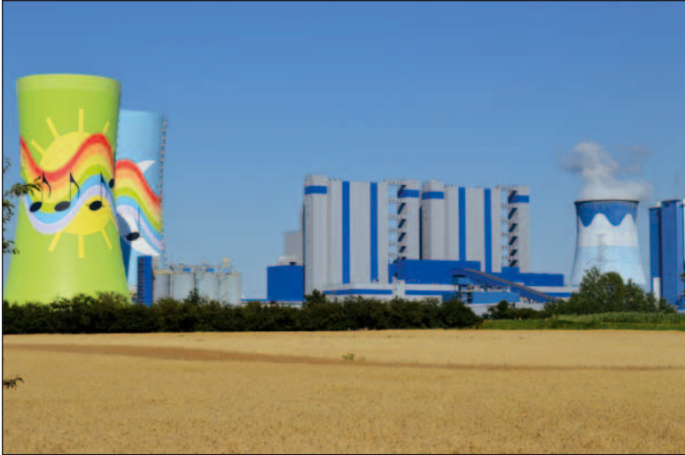
The Opole Power Station and the farmlands in Dobrzeń Mały, photo by Mirosław Marczyk, 2018
