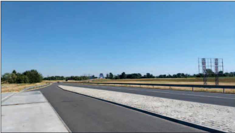
Fragment of the new bypass of the village of Czarnowąsy (currently part of Opole), photo by Mirosław Marczyk, 2018
