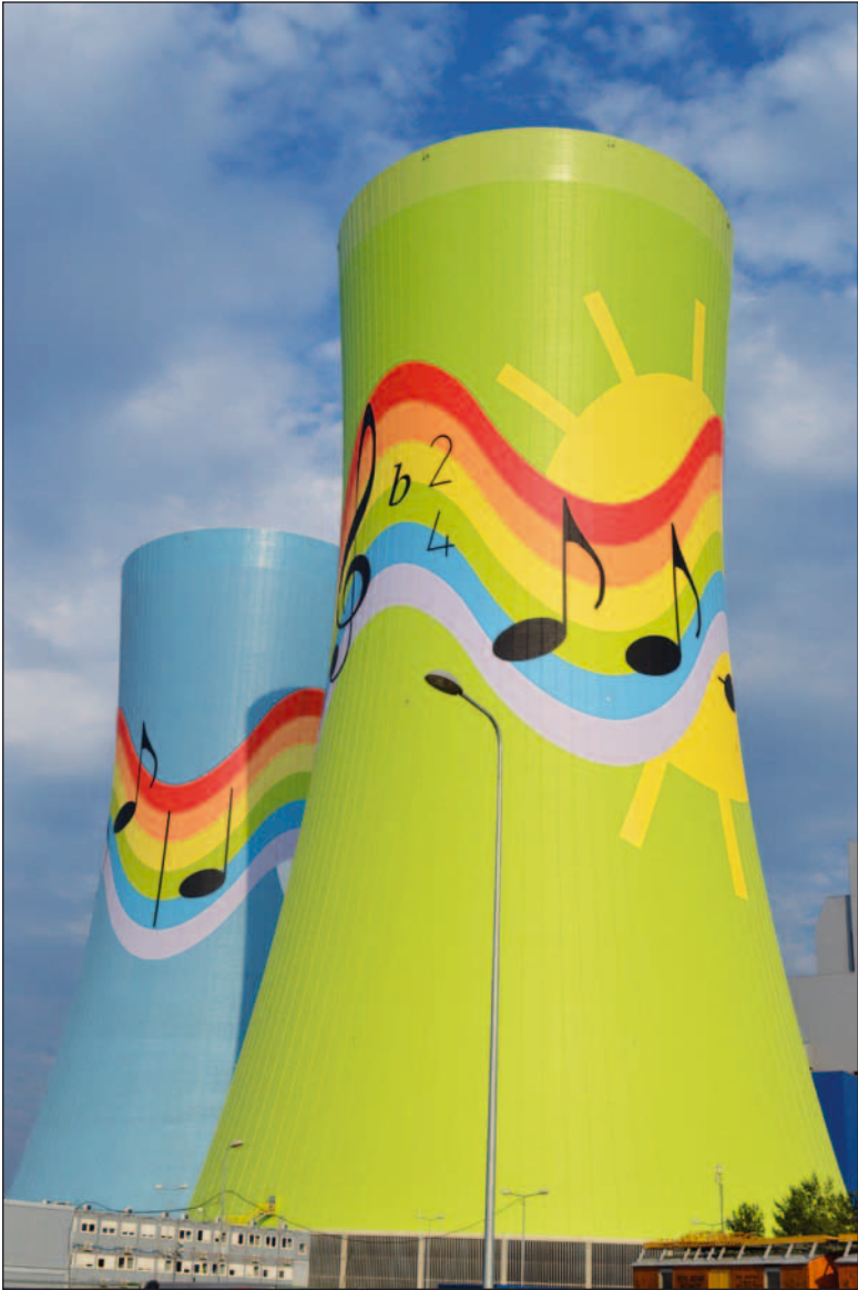
The Opole Power Station, new cooling towers, photo by Mirosław Marczyk, 2018
