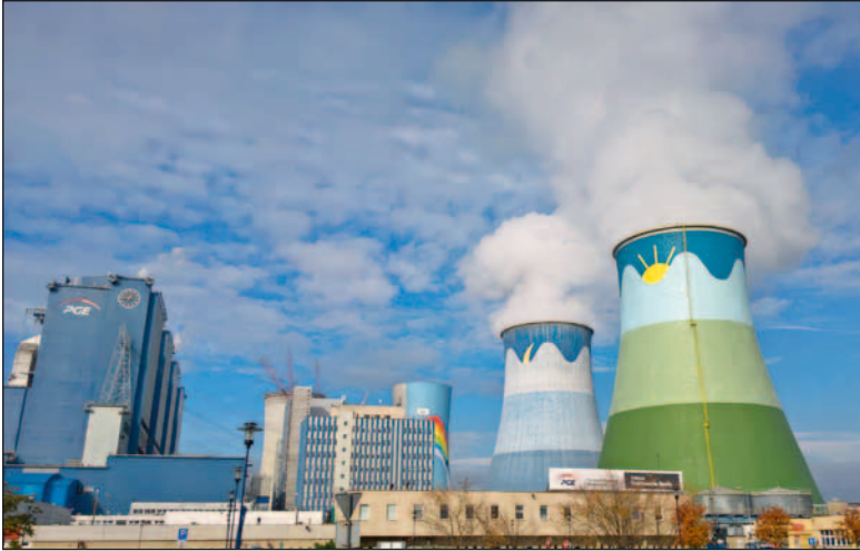
The Opole Power Station, photo by Konrad Górný, 2016
